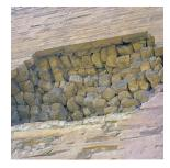
Left: A gash in the side of one of the pyramids shows a combination of irregularly cut quarried limestone blocks surrounded by tight-jointed, cast-in-place geopolymer blocks. Right: Curved, perfectly aligned joints between these backing blocks are evidence of the blocks being cast in place rather than poured. Below: A ground level block in front of the Great Pyramid of Khufu includes an irregular lip at the bottom. This lip indicates that the block was cast
